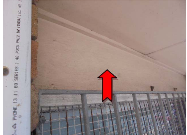
Photo 2. Exterior, north elevation, Infill panels – asbestos-containing fibre cement sheeting.
