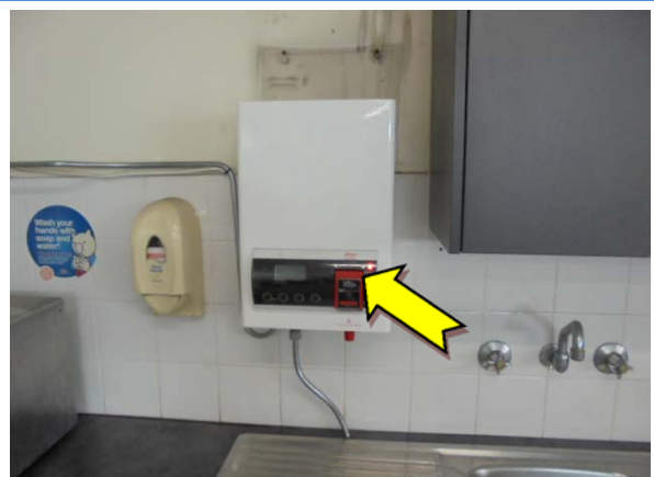
Photo 6. Interior, ground level, kitchen, hot water heater – suspected SMF internal insulation.
