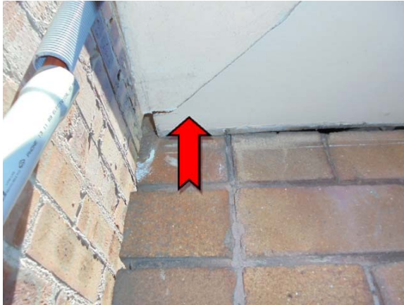
Photo 1. Exterior, north north-eastern elevations, eaves –asbestos-containing fibre cement sheeting.
